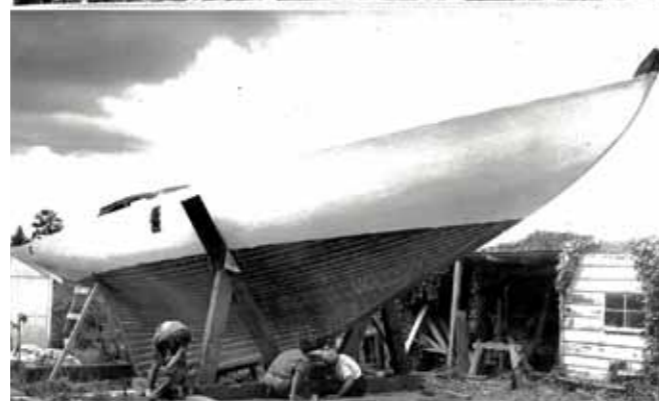
Top: Leda's hull with fore-and-aft planking completed over the inside diagonal skin. Lower: The yacht is slid around from her building site to await the low-loader.
